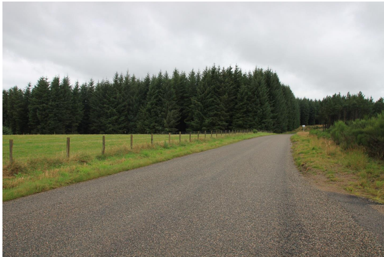
Photographic Figure 6.14: Illustrative Photograph looking north-north-westwards north of Pitchaish illustrating the forestry enclosure along this stretch of the C13E route.
